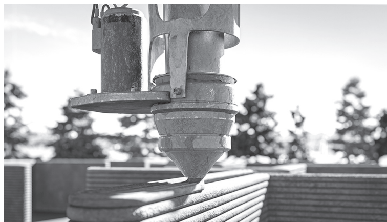
Figure 6: The nozzle of the 3D-printing robot's arm as it constructs the wall of a house
